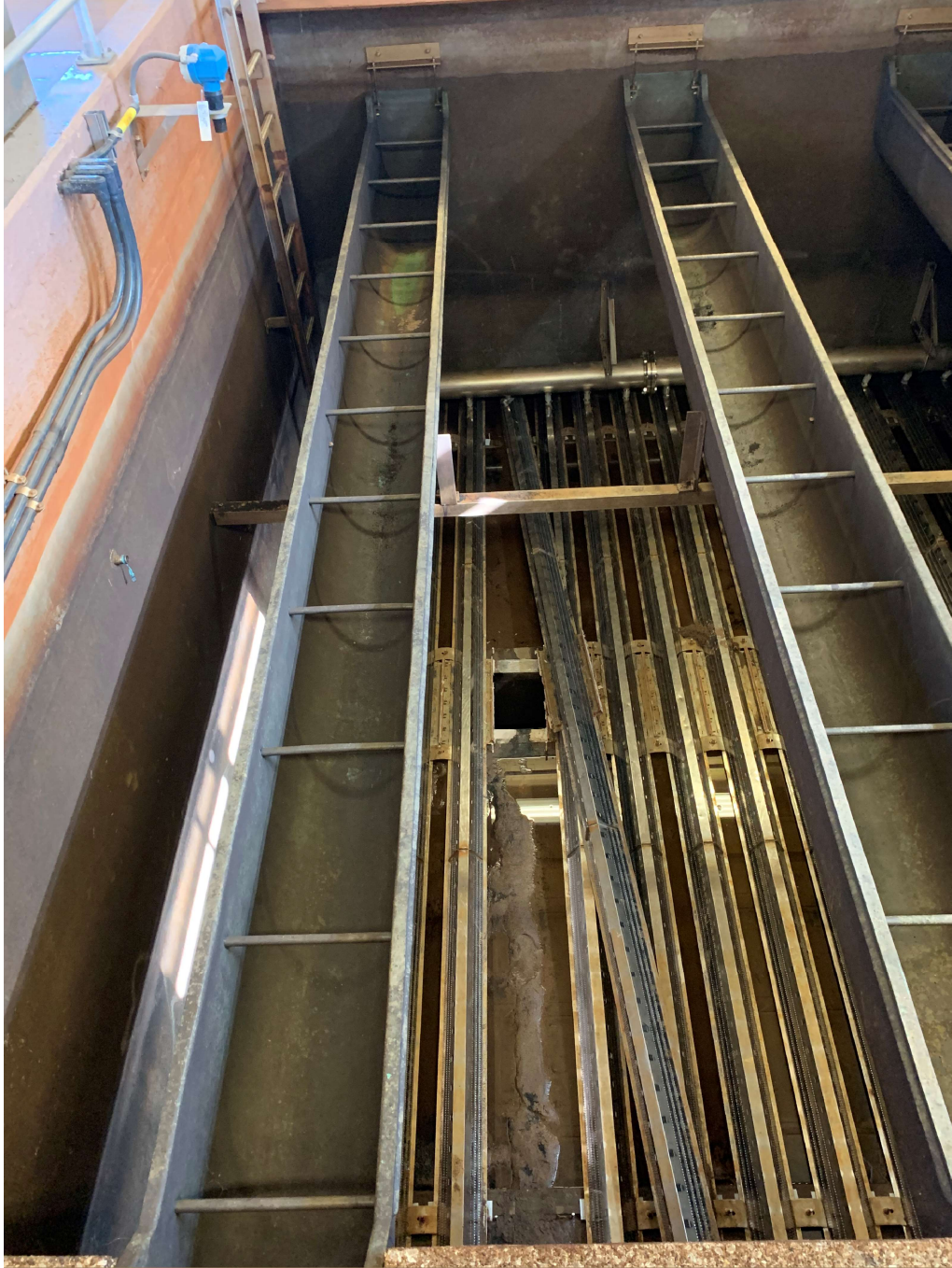
LLWTP Filter 4: Damaged Underdrain, 08/2024
