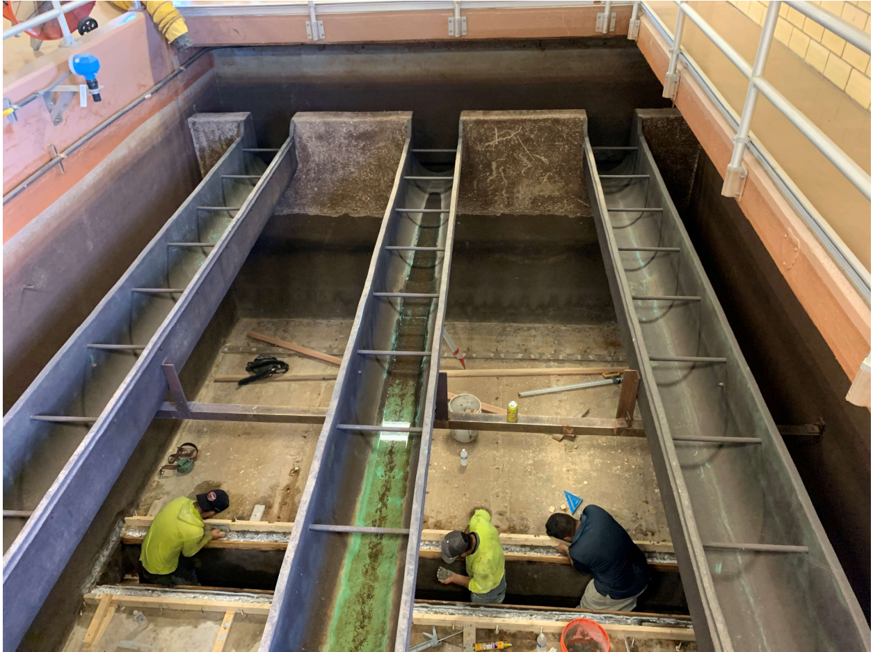
LLWTP Filter 4: Repairing Underdrain Connection, 08/2024
