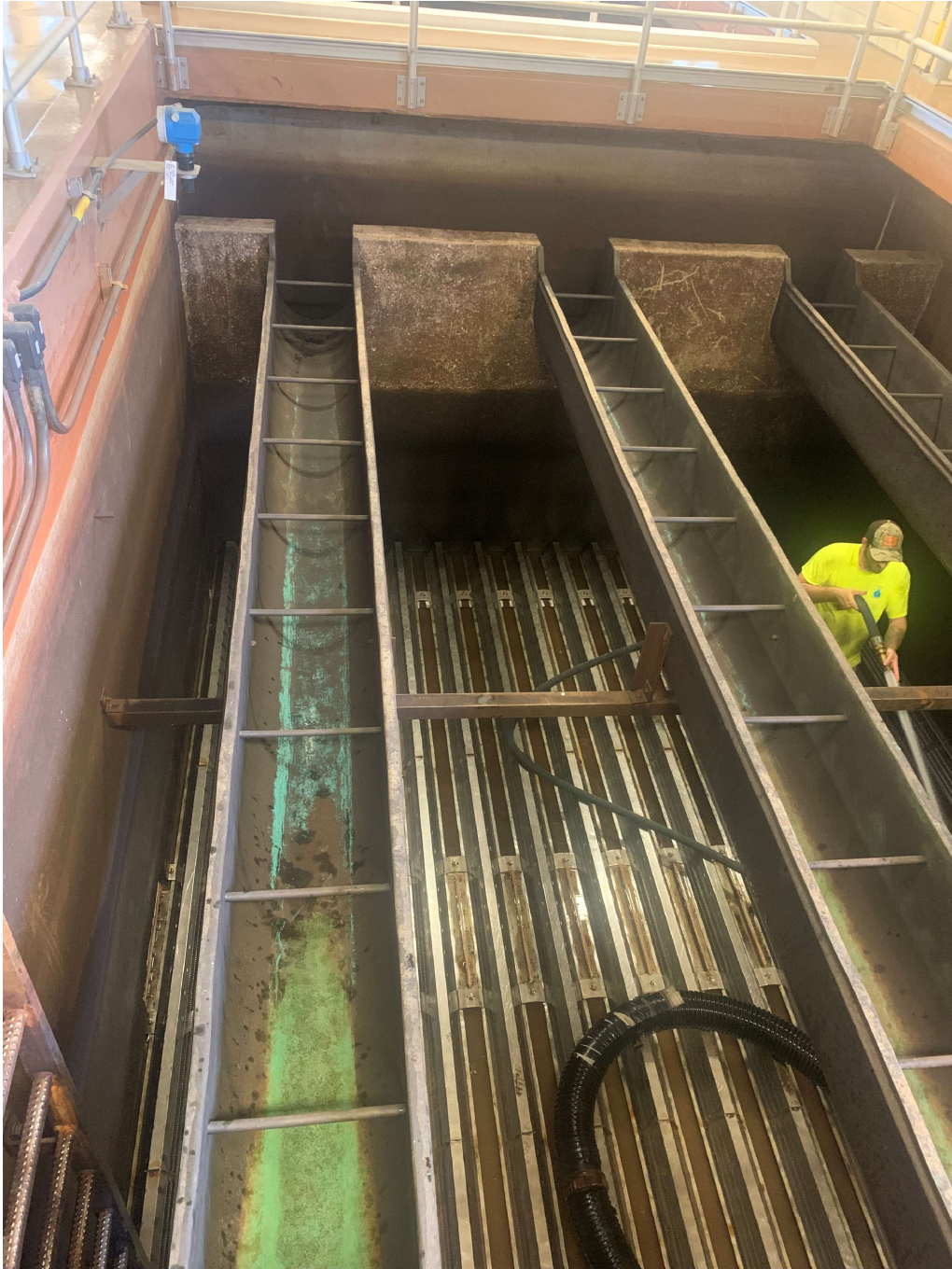
LLWTP Filter 4: Removing Filer Media, 08/2024
