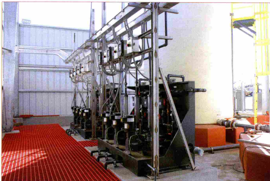
Figure 3 – Ferric Chloride Feed Pump Skid
