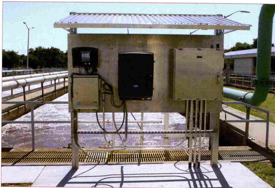
Figure 5 – Phosphate Analyzer at Aeration Basin Influent
