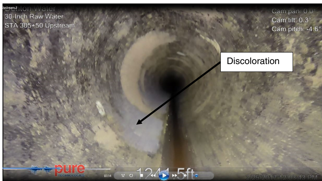
Figure 3.10: Pipe 2812, Large Discoloration, from invert across 9:00 position to crown, 1,245 feet from insertion (Station 305+50, Upstream, Video 3)
