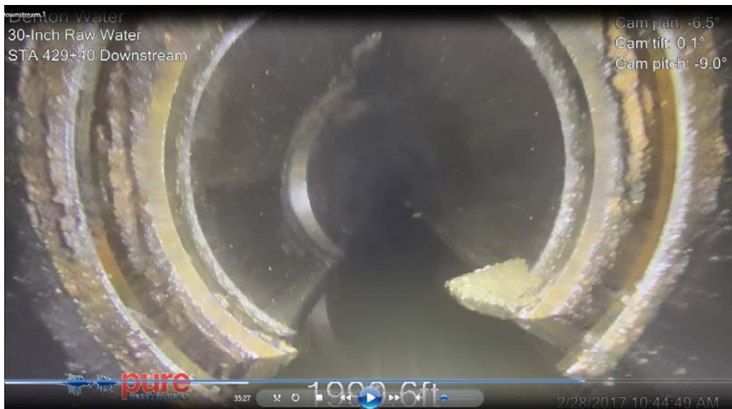
Figure 3.26: Pipe 3272, Gate valve, accumulation of debris, side outlet, 2,000 feet from insertion (Station 429+40, Downstream, Video 1)
