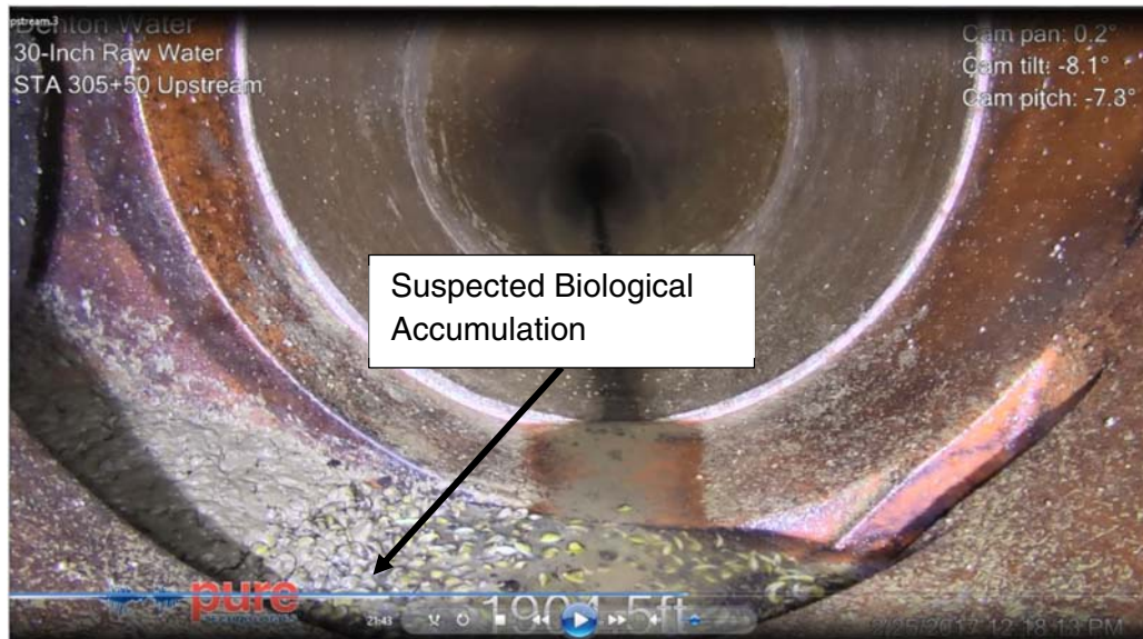
Figure 3.25: Pipe Number N/A, Gate valve, suspected biological accumulation at invert, 1,902 feet from insertion (Station 305+50, Upstream, Video 3), Laying schedules unavailable
