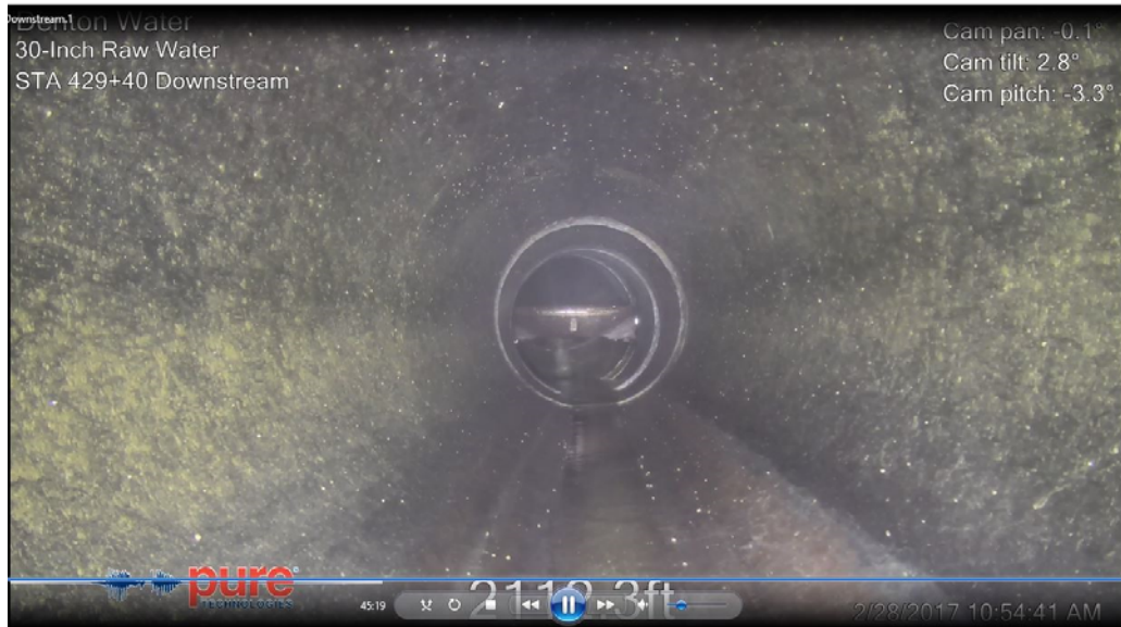
Figure 3.27: Butterfly valve, 2,125 feet from insertion towards Rapid Mix Basin (Station 429+40, Downstream, Video 1) end of inspection
