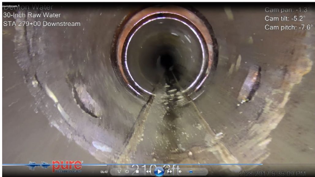
Figure 3.28: Pipe 2771, Gate valve and outlets, 210 feet from insertion (Station 279+00, Upstream, Video 1)
