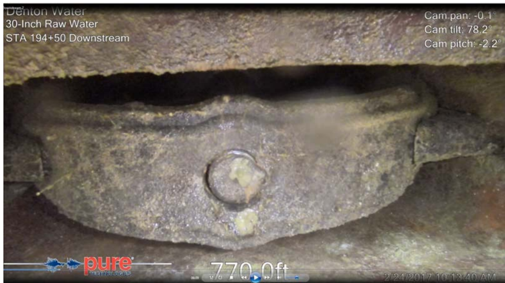
Figure 3.21: Pipe number N/A, Typical gate valve, 770 feet from insertion (Station 194+50, Downstream, Video 2), Pipe laying schedule unavailable
