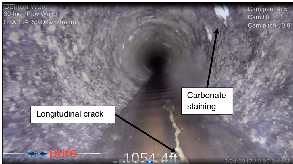
Figure 3.4: Pipe 2536, Longitudinal crack along invert, 30-feet in length, begins at 1,036 feet from insertion (Station 194+50, Downstream, Video 2)
