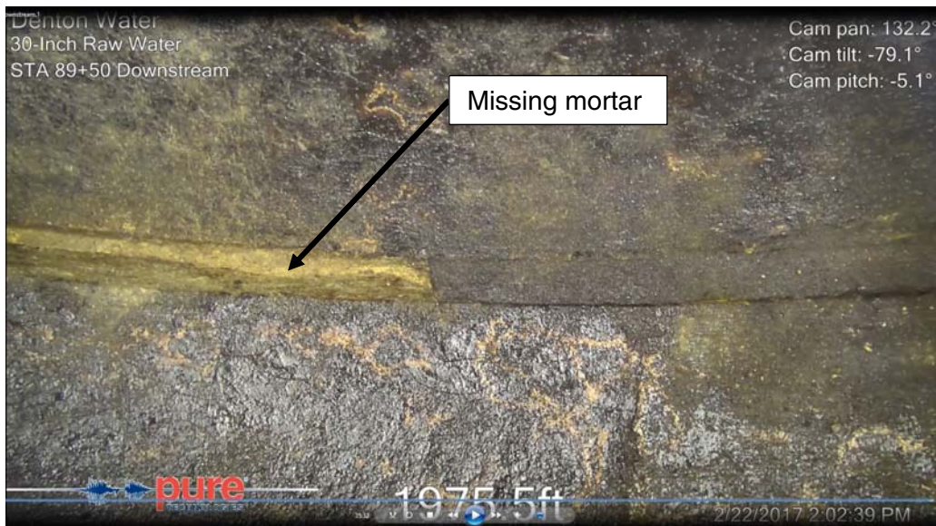
Figure 3.23: Pipe 2255, Joint missing mortar, 1,975 feet from insertion (Station 89+50, Downstream, Video 1),
