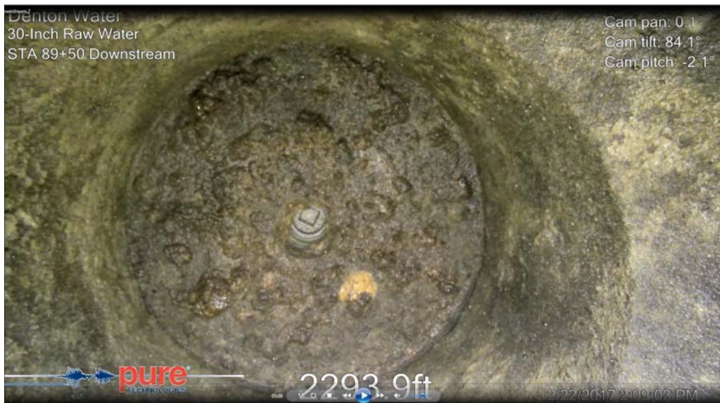
Figure 3.22: Pipe 2267, General view of top outlet, 2,294 feet from insertion (Station 89+50, Downstream, Video 2)
