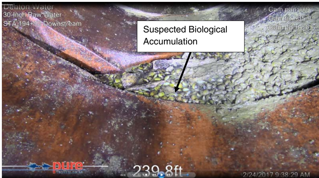
Figure 3.24: Pipe 2506, Gate valve, Suspected biological accumulation at invert, 240 feet from insertion (Station 194+50, Downstream, Video 1)
