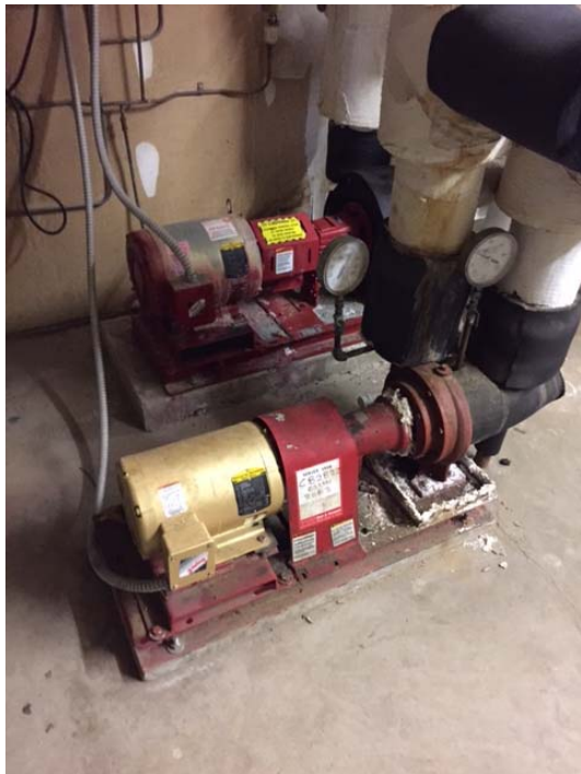
5. Chilled Water Pumps in Mechanical Room.
