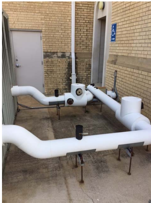
2. Chilled Water Piping.
