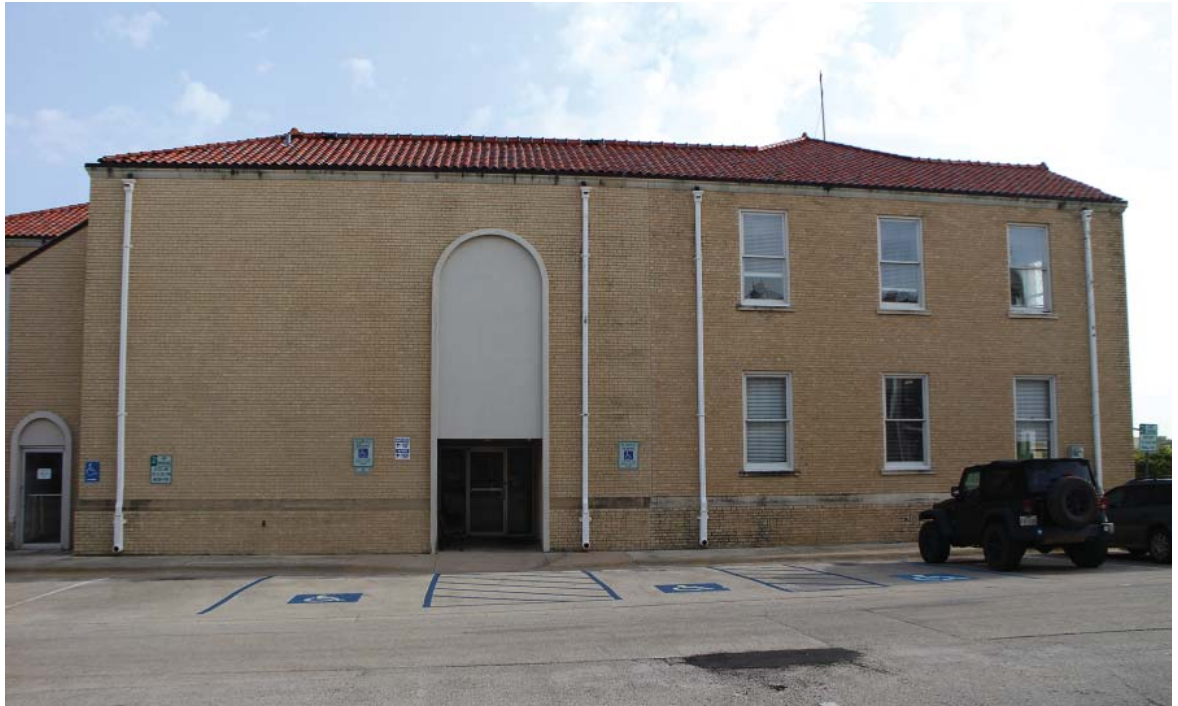
View of the south facade showing the original building at right and the addition at left. If the addition is retained, the architectural details should be improved. (Architexas 2017)
