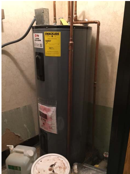
15. 50 Gallon Electric Water Heater on 1 st Floor.
