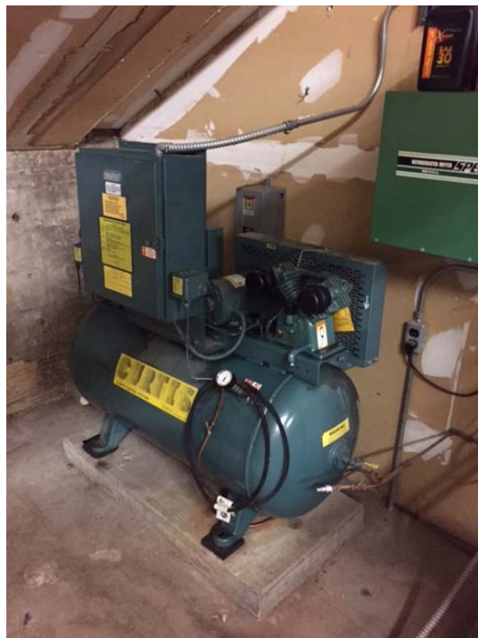
6. Air Compressor for Pneumatic Controls.
