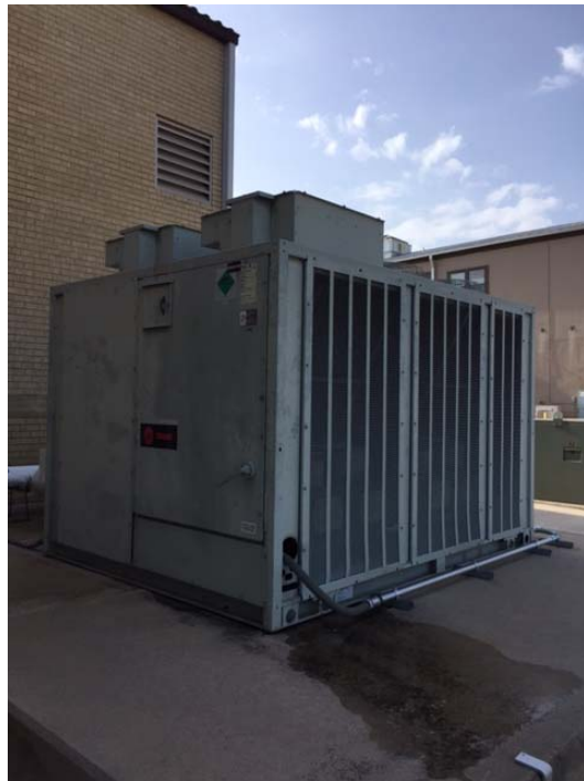
1. 60 Ton Trane Air Cooled Chiller.
