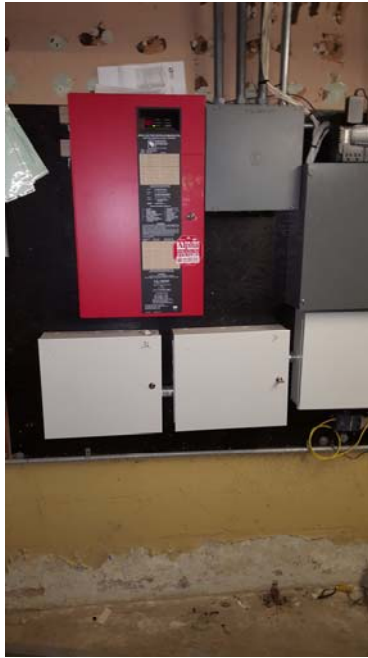
17. Fire Alarm Panel in Basement.
