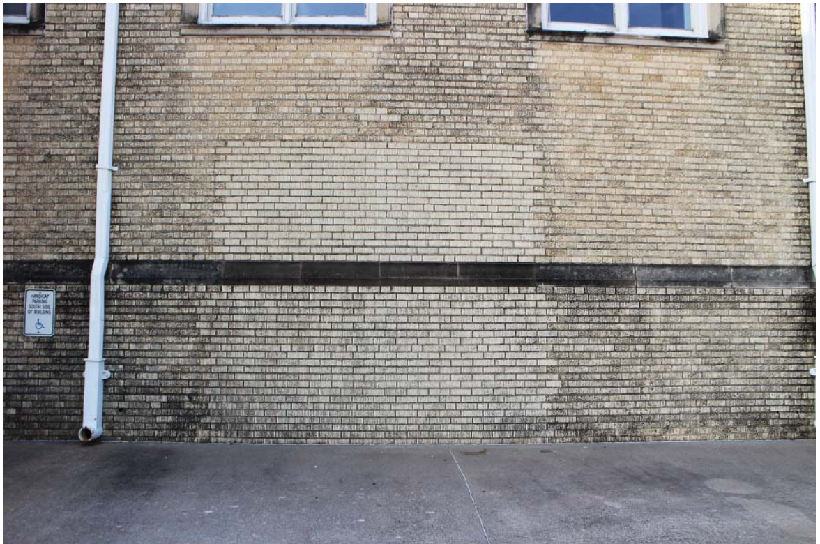
Typical masonry conditions at north elevation. Masonry needs cleaning. Brick infill at bay door location is evident. (Architexas 2017)
