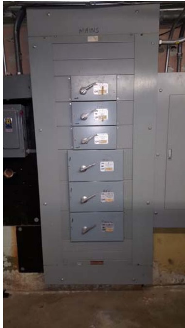
10. Main Switchgear in Basement.
