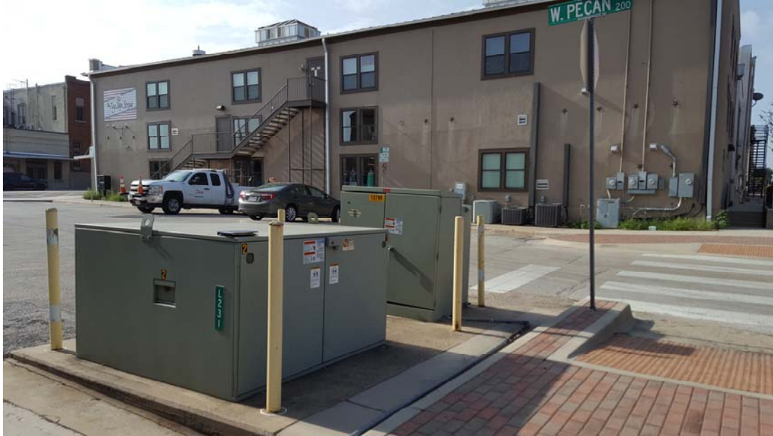
9. Utility Company Switch and Transformer for Building.
