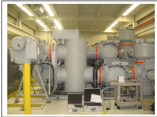
Typical GIS Equipment Section (138kV Circuit Breaker, Bus, Switches, and other Hardware)
