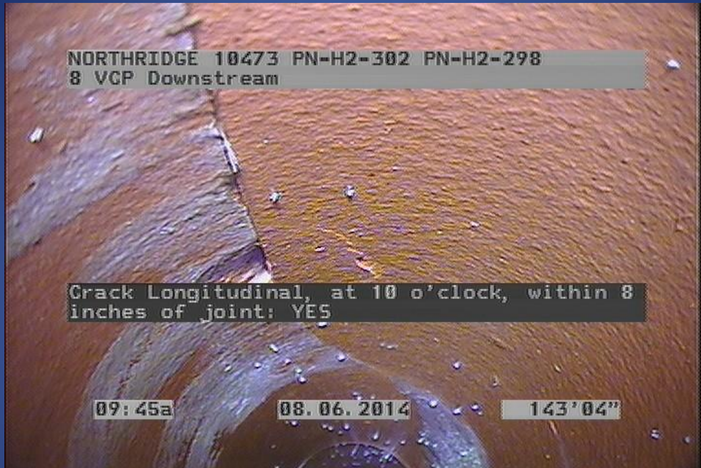
CCTV picture of fracture allowing infiltration.
