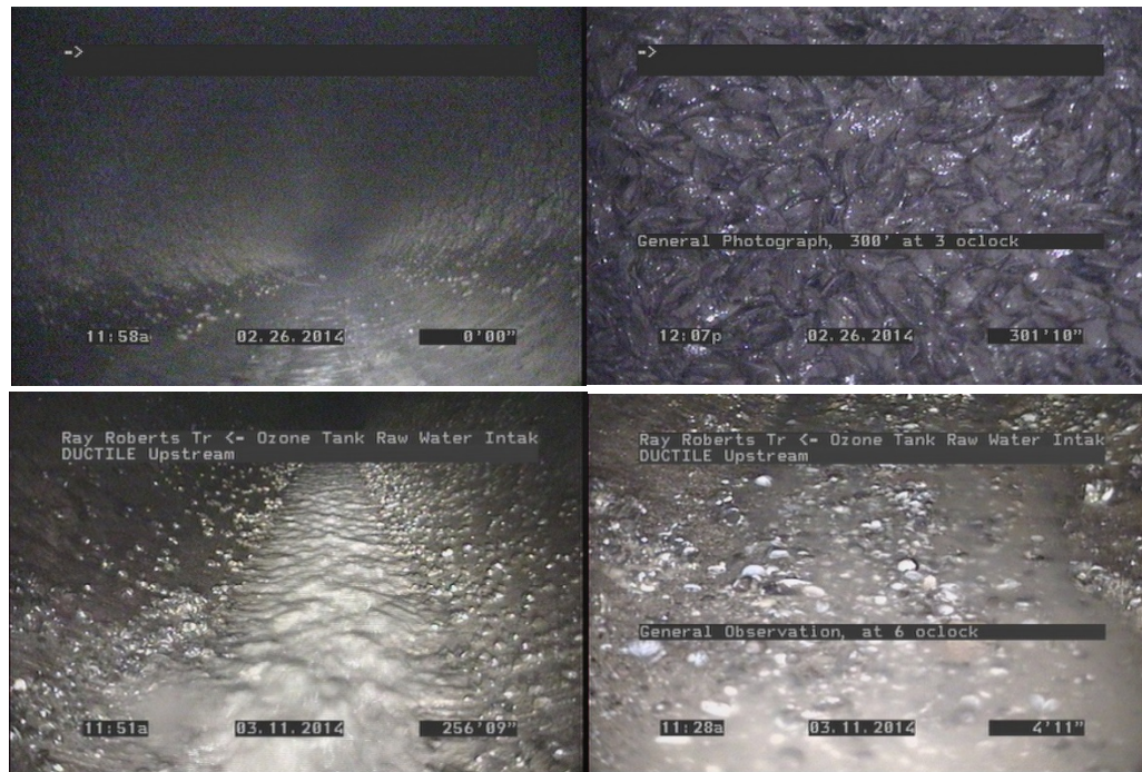
Figure 2-8: Zebra Mussel Shells in the City of Denton Raw Water Pipelines (March 11, 2014).
