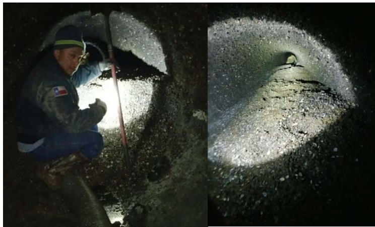
Figure 2-13: 50-80% Blockage of Mussel Shells in the Low Section of the 60" RRWTP Raw Water Pipeline Downstream of Ray Roberts Lake (February 2015)
