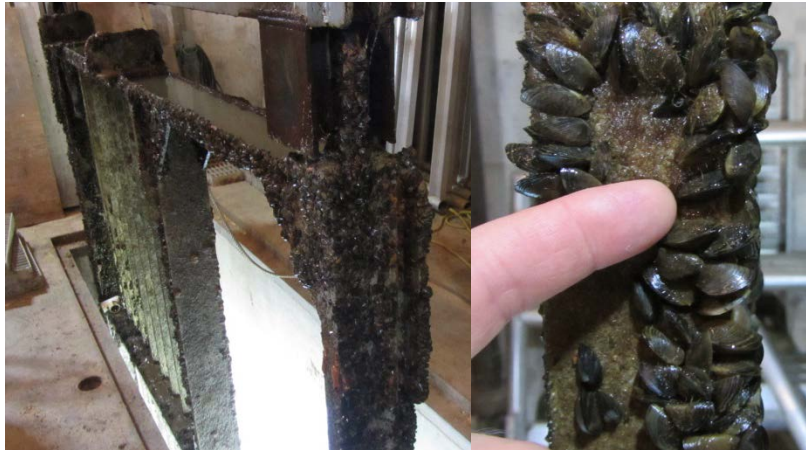
Figure 2-7: Zebra Mussel Infestation of the Ray Roberts Lake USACE Outlet Trash Racks (October 31, 2013)
