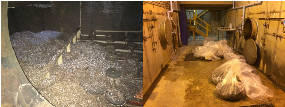
Figure 2-12: Zebra Mussel Observations and Removal in the Ozone Contactors at the RRWTP (January 2015)
