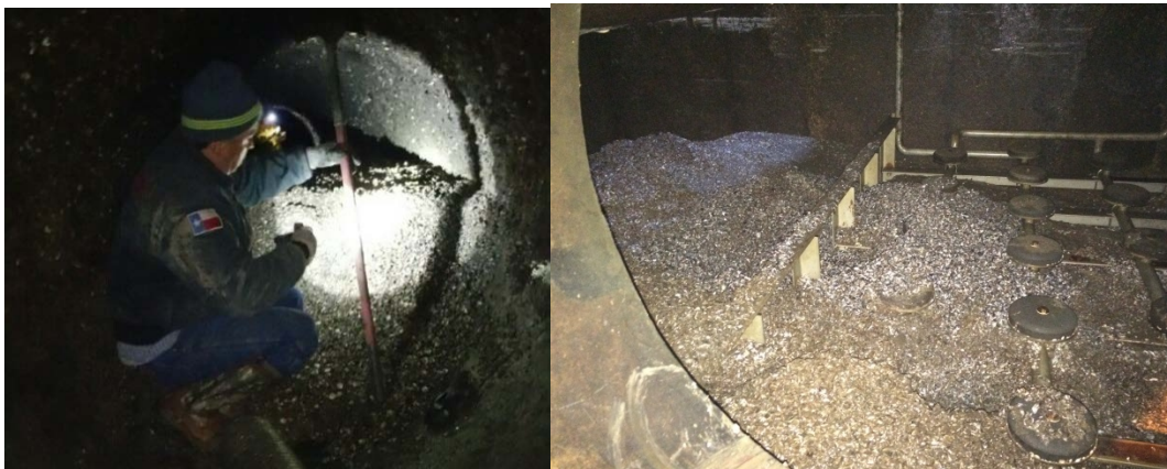
Figure 2-3: Zebra Mussel Shells in the COD Raw Water Pipeline and Ozone Contactors
