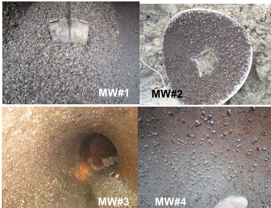
Figure 2-11: Zebra Mussel Observations at the Location of RRWTP Raw Water Manways (December 2014)
