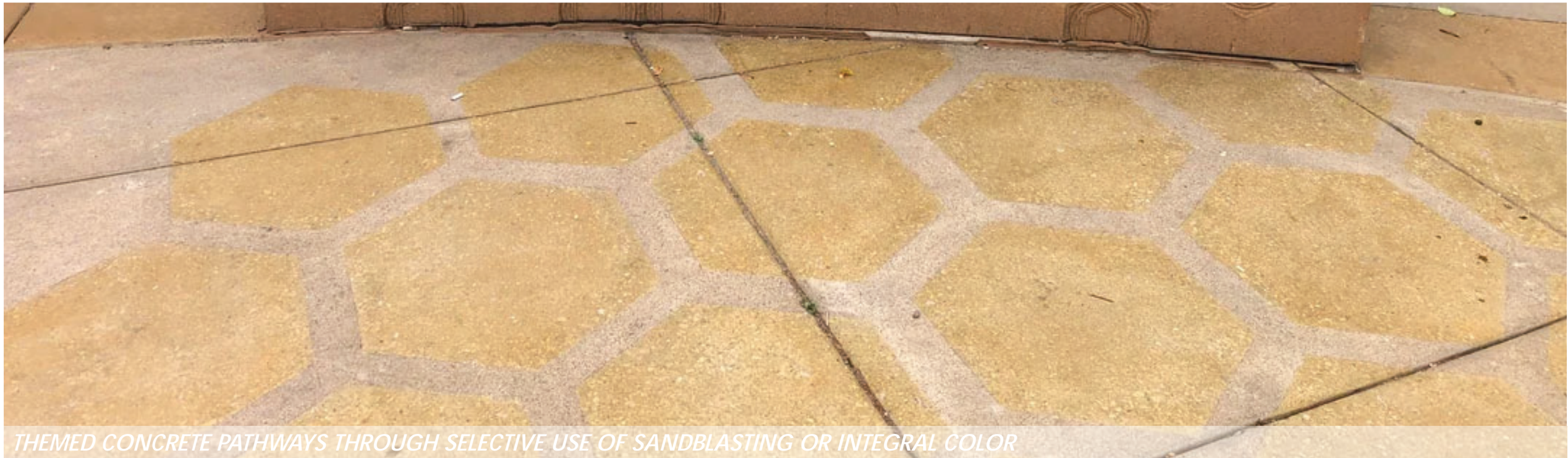
THEMED CONCRETE PATHWAYS THROUGH SELECTIVE USE OF SANDBLASTING OR INTEGRAL COLOR
