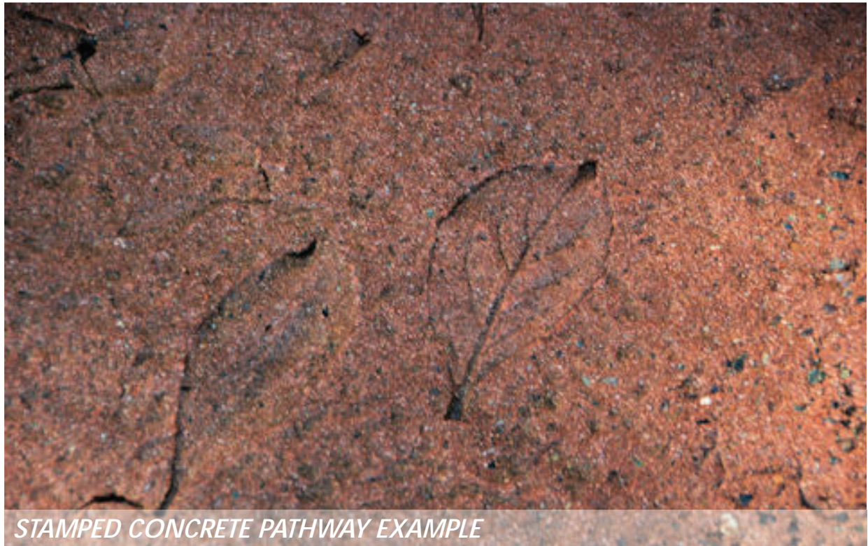
STAMPED CONCRETE PATHWAY EXAMPLE
