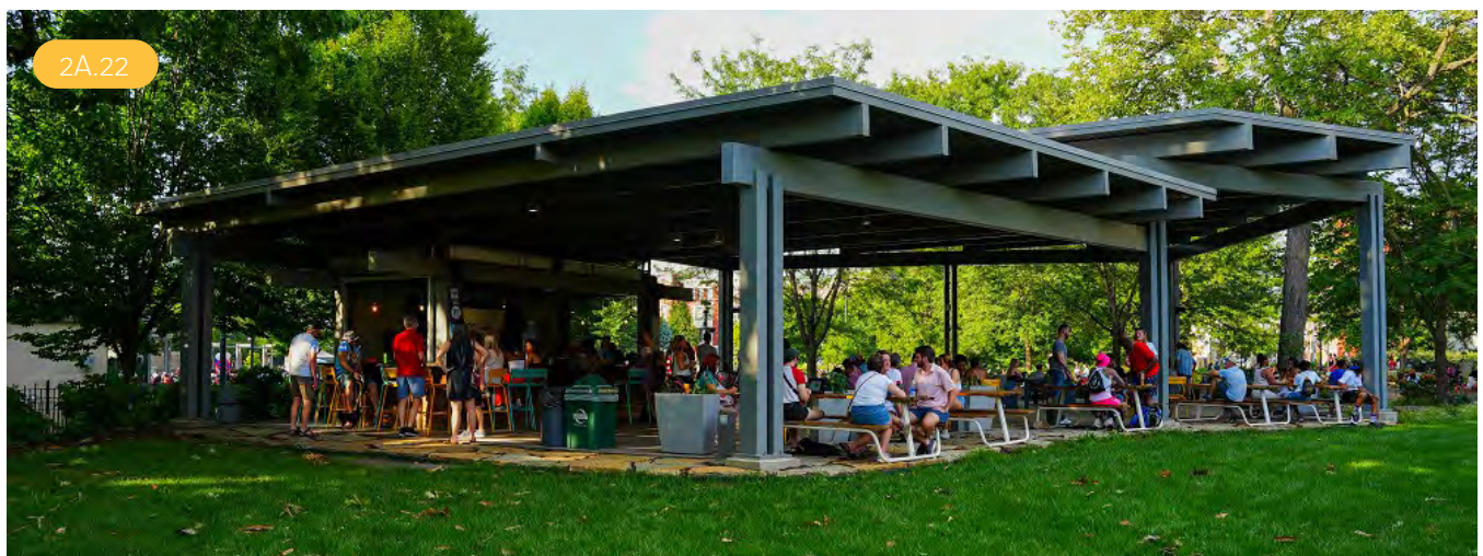
The Porch in Cincinnati's Washington Park is a great example of a community rest stop in the park, where folks can drop by for a soda, beer, wine, or snack, and sit in the shade surrounded by nature. Facilities like this can operate via contracted vendor, City-operated vending, or seasonal/rotational vending. Image Credit Cincinnati Center City Development Corporation.
