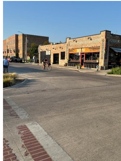
(B) Missing crosswalk at Industrial St.
