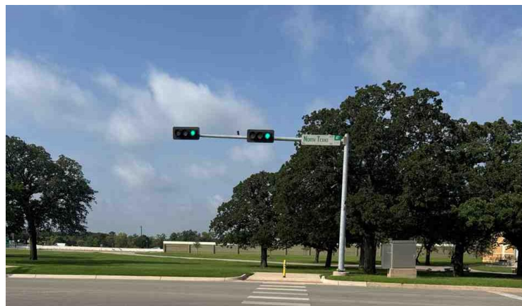
Figure 14 – Example of Missing Retroreflective Backplates
