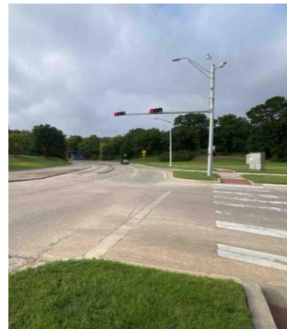
Figure 6 – Example of Faded Pavement markings
