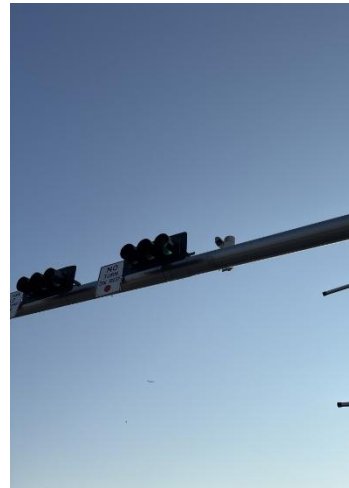
Figure 9 - Example of Missing Retroreflective Backplates
