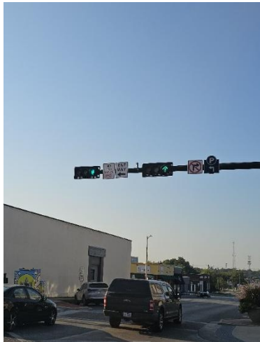
Figure 9 - Example of Missing Retroreflective Backplates
