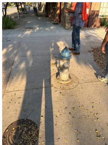
(A) Fire hydrant on the north side of the corridor, east of Oakland St
