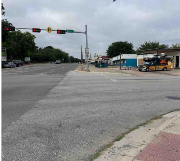
Figure 11 – Example of Missing Crosswalks
