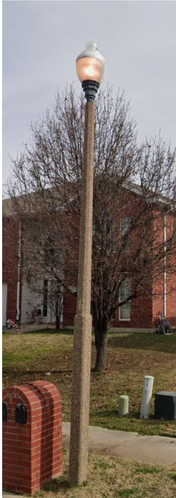
Figure C.1: Residential Lighting – 20-ft. concrete aggregate pole with post-top luminaire
