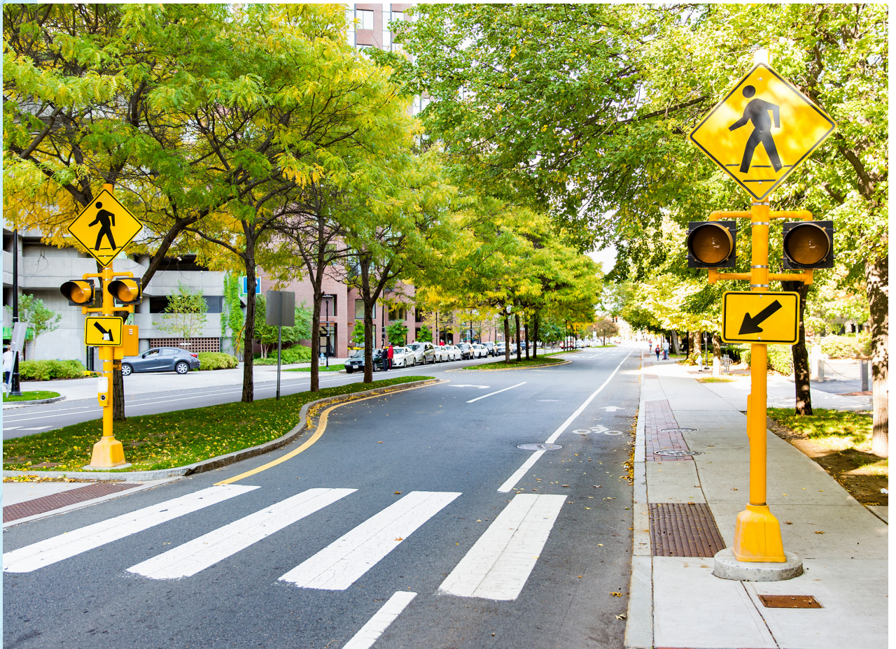
Figure 4.10. Mid-Block Crosswalk Example
