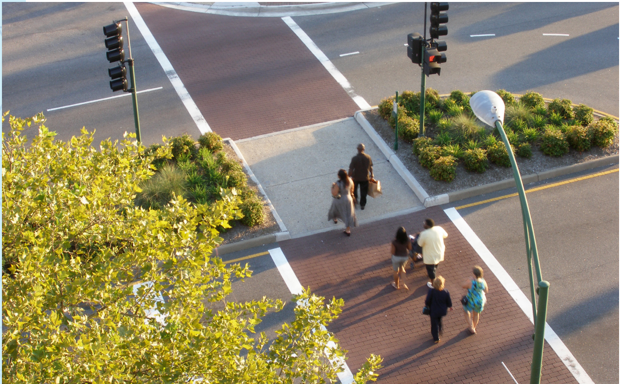
Figure 4.1. Raised Medians and Pedestrian Refuge Island Example
