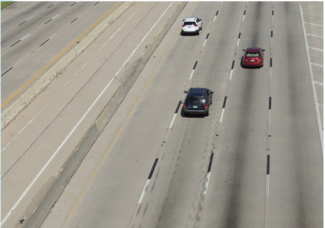
Figure 4.11. High Contrast Lane Markings Example
