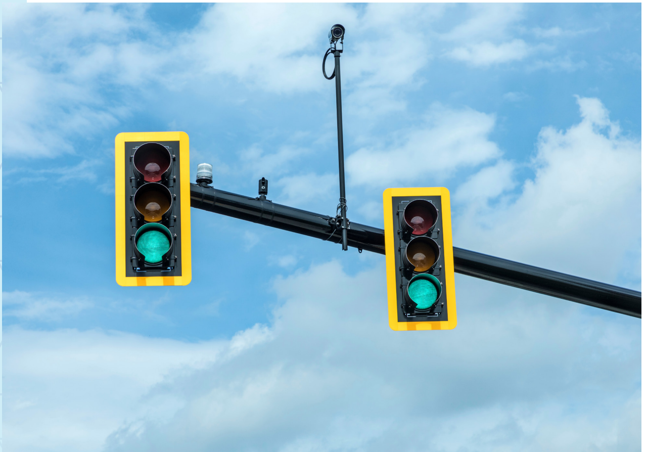
Figure 4.12. Retro-Reflective Backplates Example
