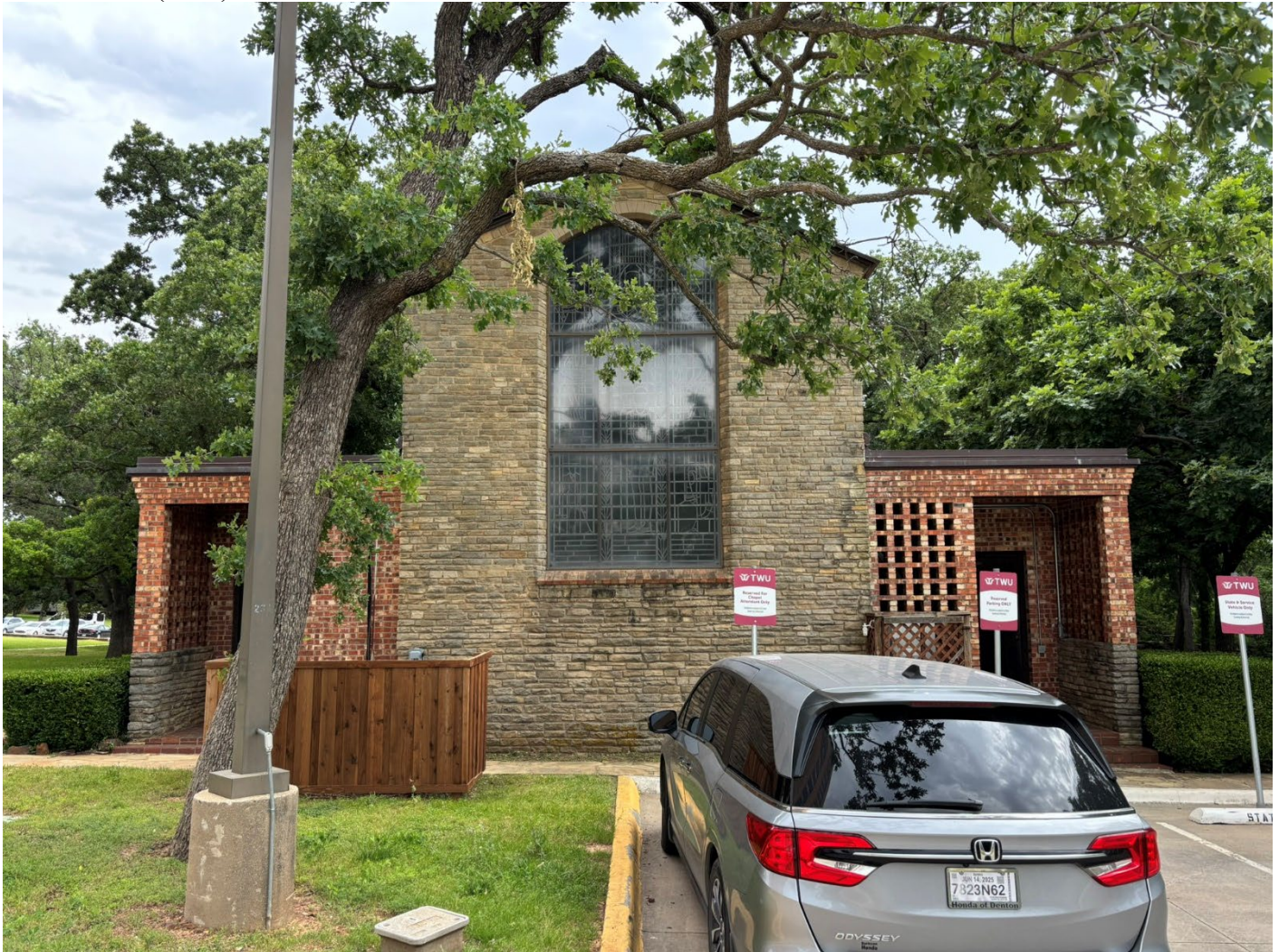
Photo 7: Rear (north) elevation
