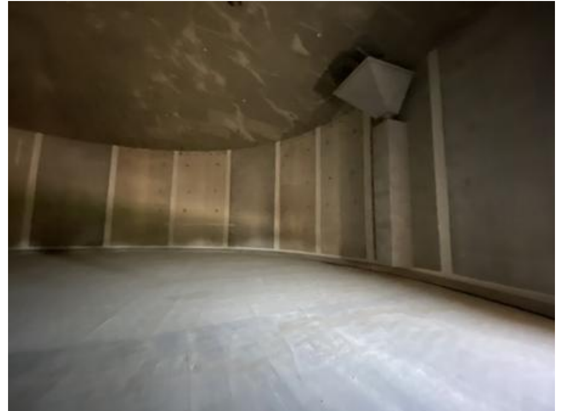
Clear well improvements
