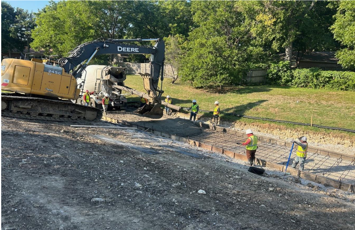
City of Denton Excavator
