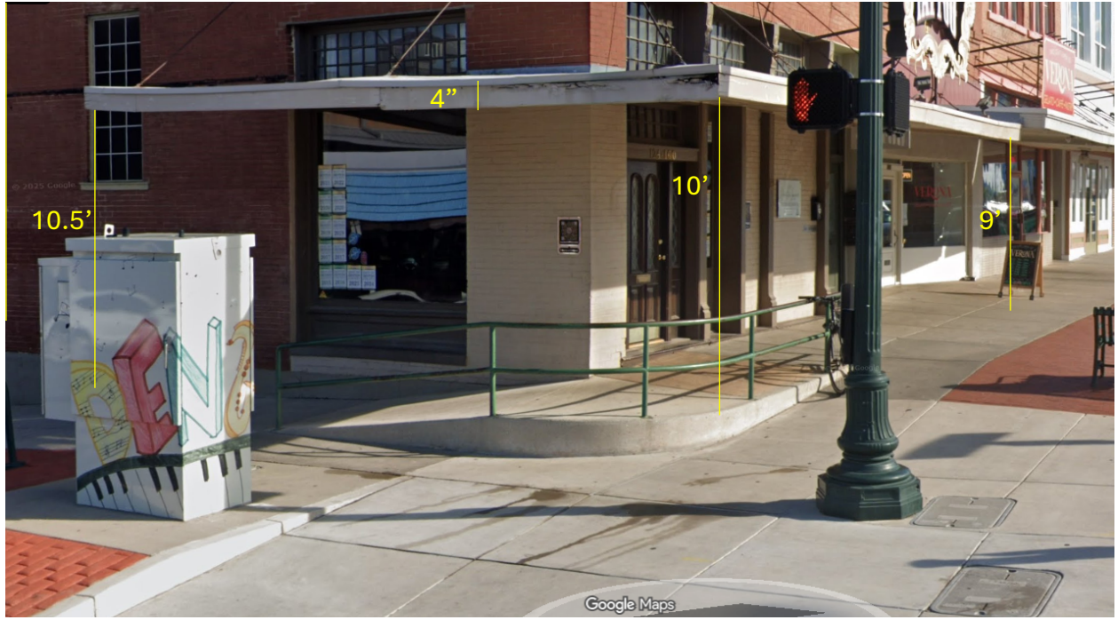
Area of repairs
