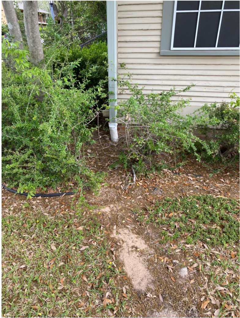
New Drainage System
