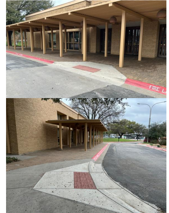
Civic Center ADA Approach Project Cost: $ 16,391.02
