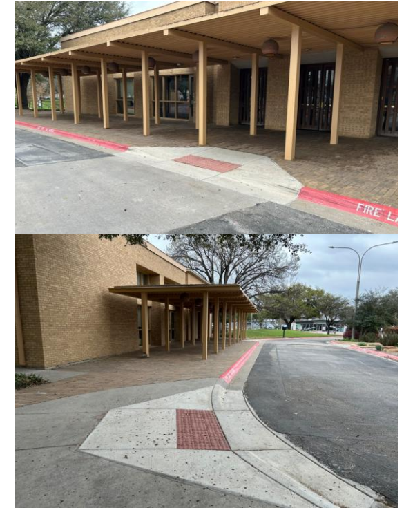
Civic Center ADA Approach Project Cost: $ 16,391.02
