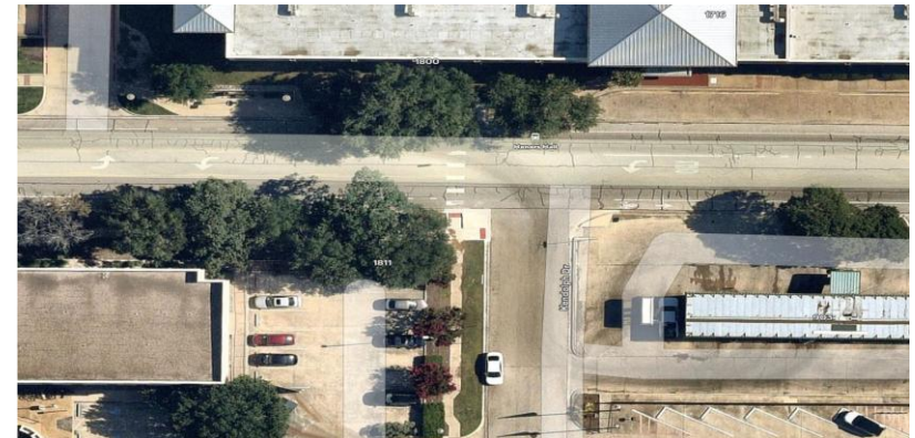
Kendolph Drive and Eagle Road (Before and After Installation)
