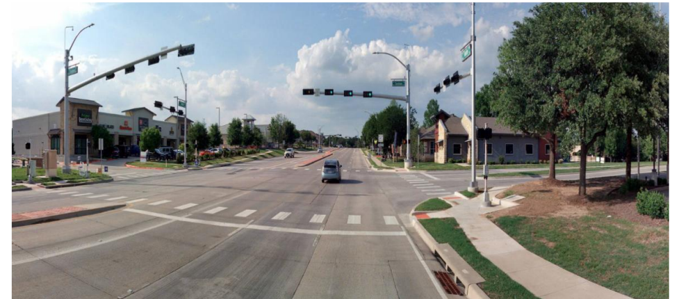
Teasley Ln at Sundown Blvd Intersection (Before and After Installation)
