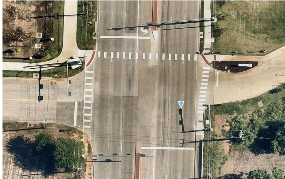
Duchess at Loop 288 (Before and After Installation)
