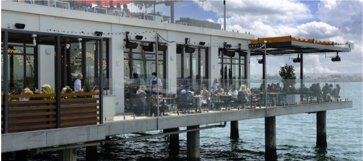
Example of deck-over water feature
