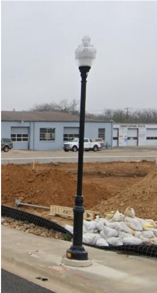
Figure C.4: Historic District Lighting – 12-ft. concrete aggregate pole with post-top luminaire
