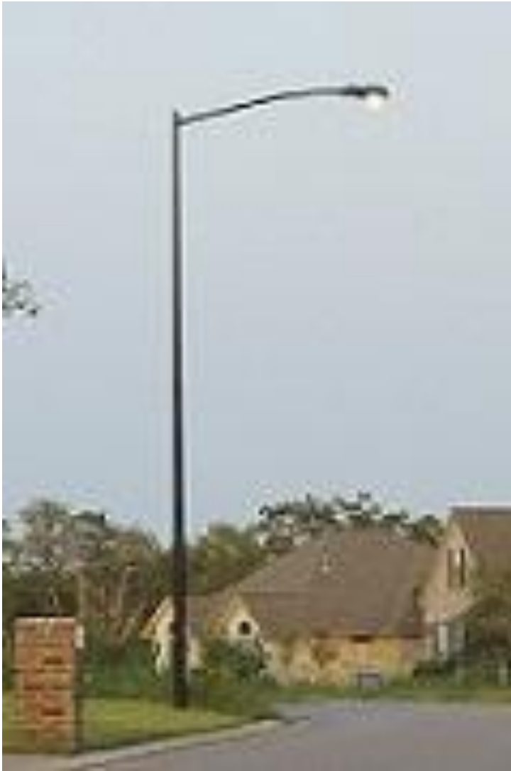
Figure C.5: Alternate General Streetlighting – 35-ft. dark gray steel pole with single or double mast arms and new cobra head luminaire.
