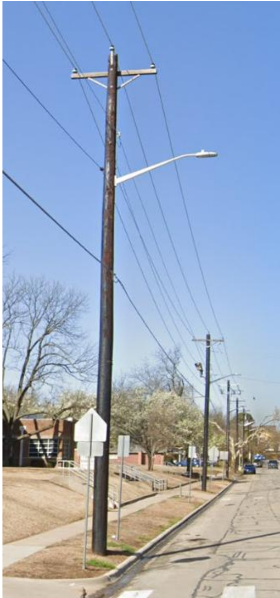
Figure C.2: General Street Lighting – Wood (distribution) pole with single-mast arm and cobra head luminaire
