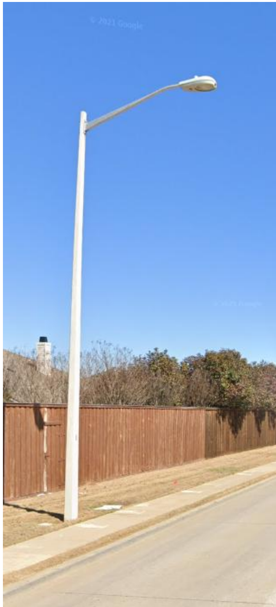
Figure C.3: General Street Lighting – 35-ft. white concrete pole with single or double-mast arms and cobra head luminaire
