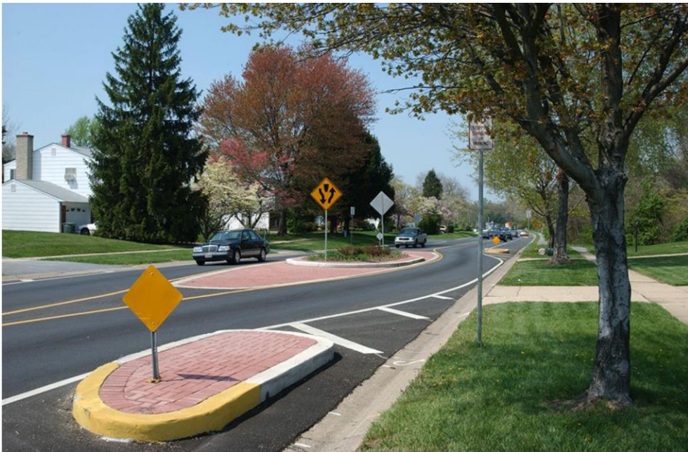
Chicane on a residential street. Source: NACTO
