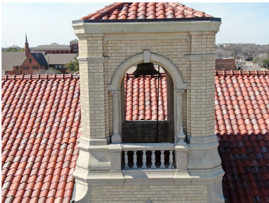
Bell tower cast stone balustrade, east elevation, missing urn
