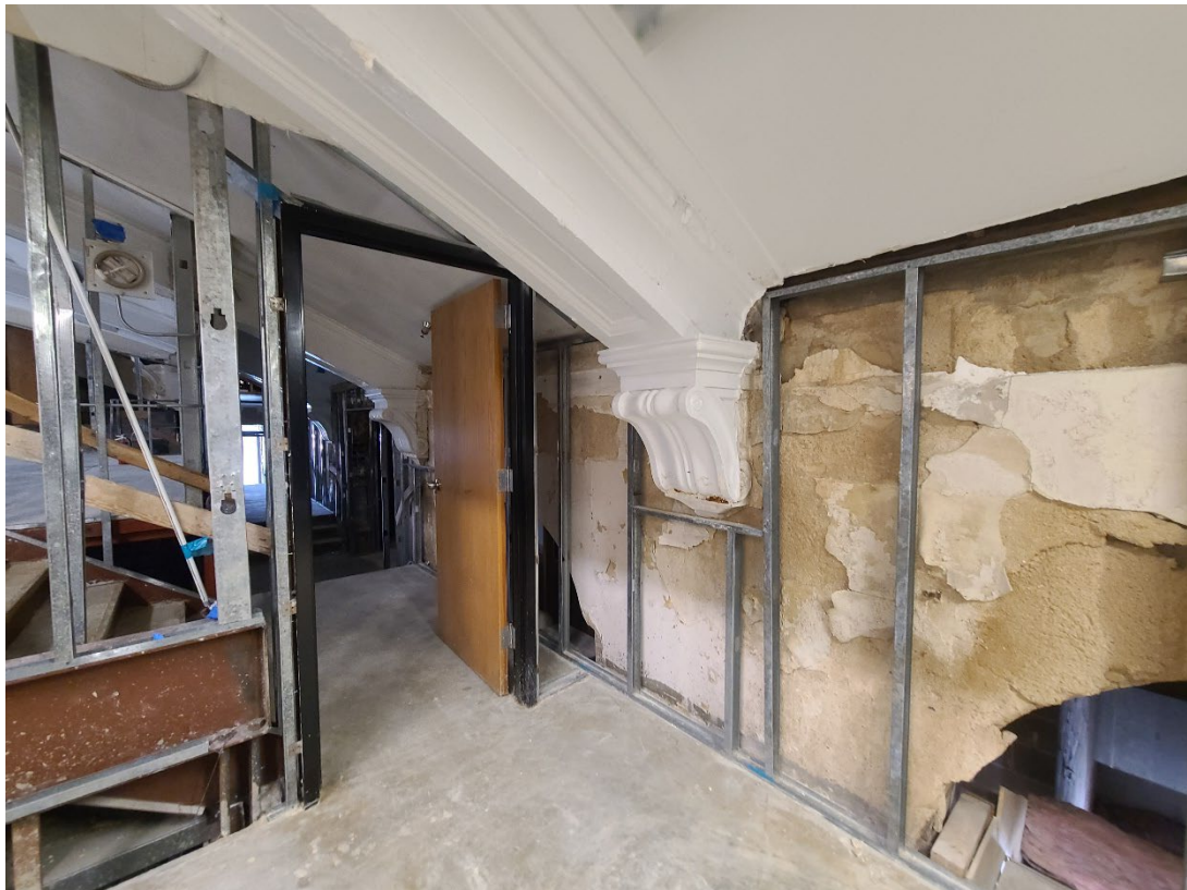
Level F original south wall, masonry opening, ceiling plaster work, infill floor
