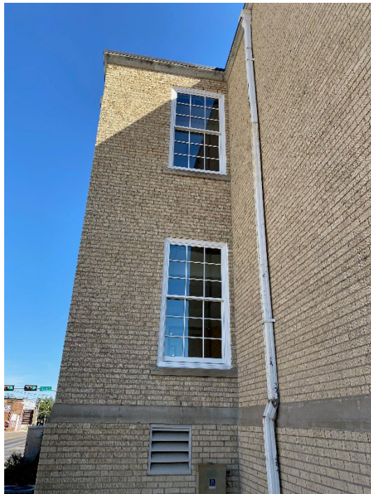
Existing Type F and cast stone surround
