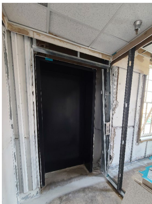
Level C North elev. Door in former window opening
