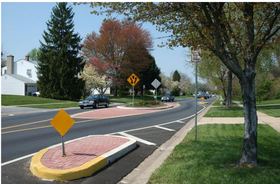
Chicane on a residential street. Source: NACTO
