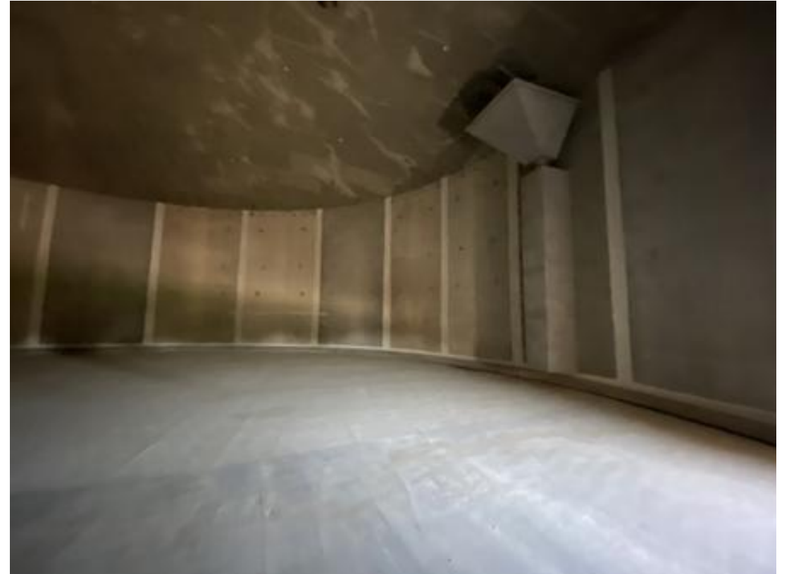
Clear well improvements
