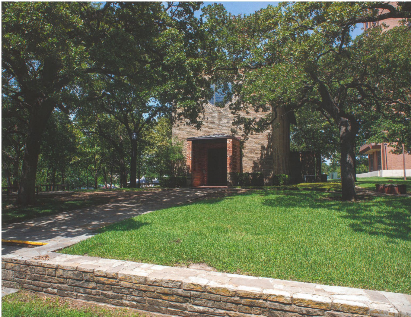
Photo 1: Front (south) elevation showing retaining wall.
