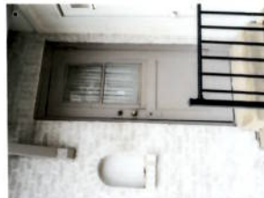
1009 Back Door (east side)-0001025
