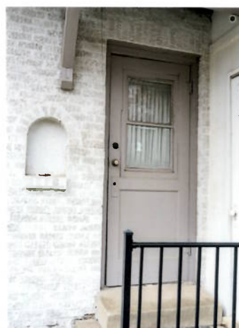
1009 Back Door (east side)-0001025
