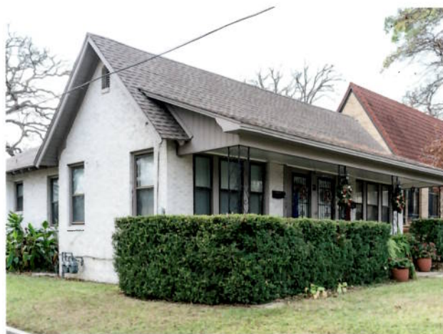
Front 3-4, East Side-0001036
