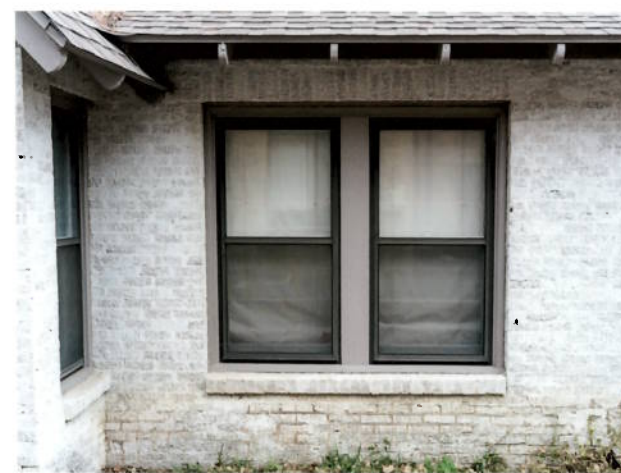
1011, Dining, East Side close-up-0001011
