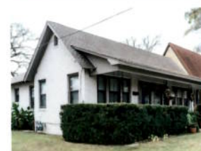
Front 3-4, East Side-0001036
