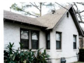
1009 East Side (looking north)-0001035
