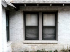
1011, Dining, East Side close-up-0001011
