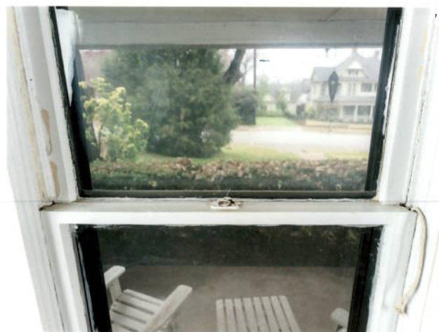
Interior, 1011, Living Rm, North Facing, Detail-0001082
