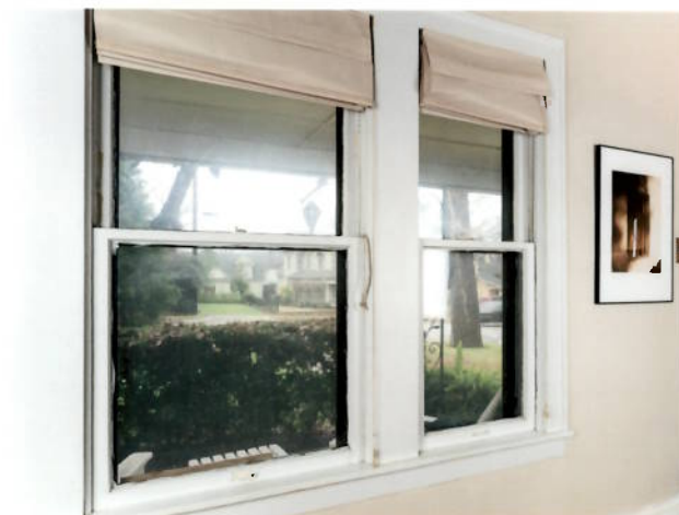
Interior, 1011, Living Rm, North Facing-0001077
