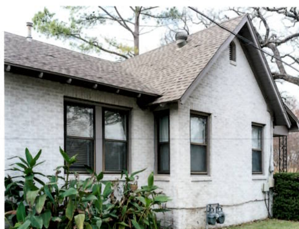
1009 East Side (looking north)-0001035
